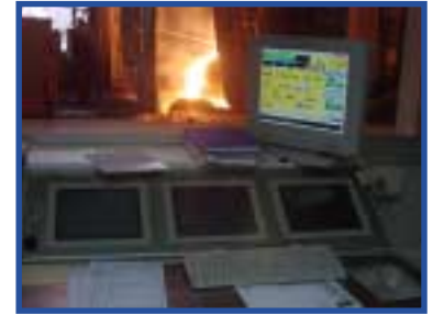
Main Control Desk
