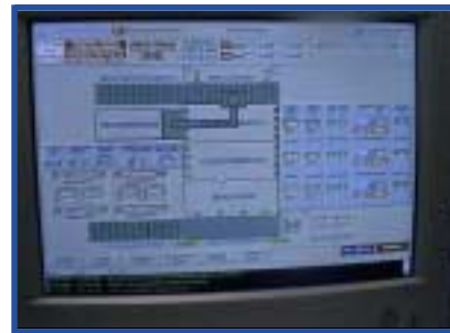
Reheating Furnace Mask
